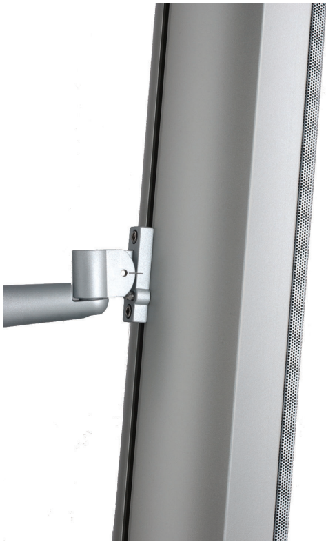
Detail mounting bracket
